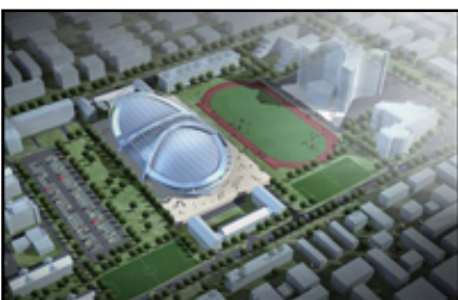
Beijing Institute of Technology Gymnasium
